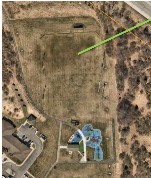
Dark Area Indicates Poor Drainage (2022)
