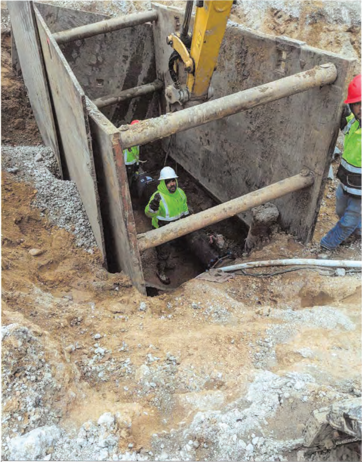
Watermain repair along Grand River where directional drill damaged watermain
