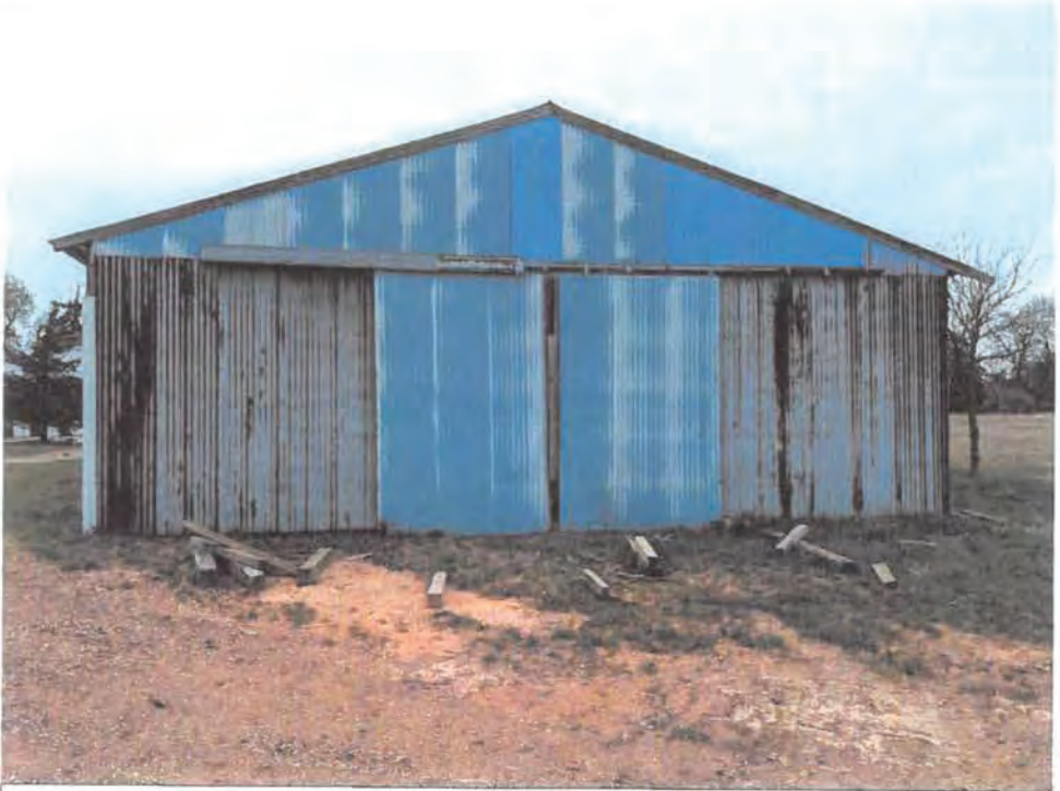
Picture 4 – Rear of Larger Pole Barn Looking South
