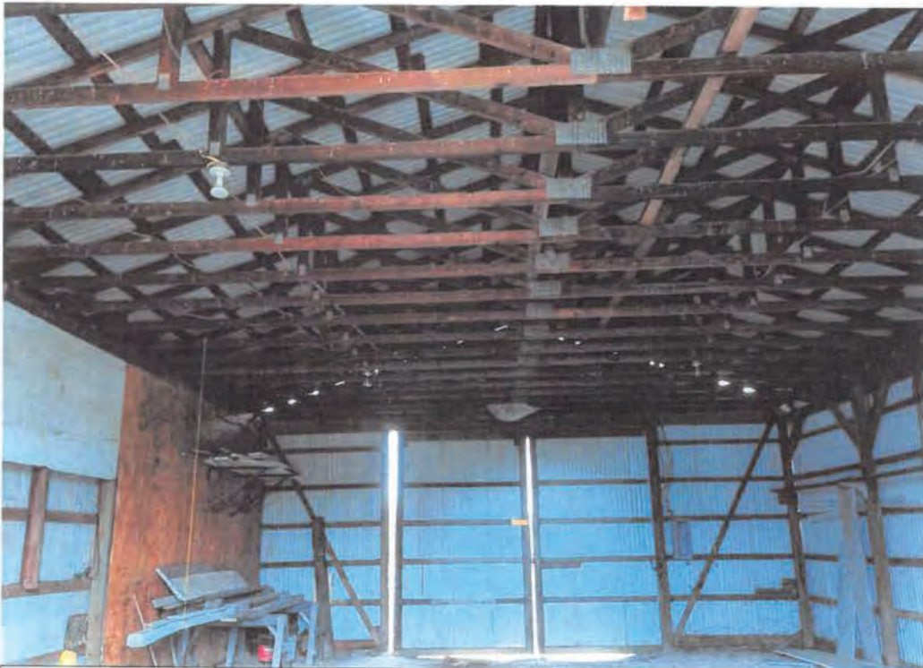
Picture 11 – Interior Smaller Pole Building Looking West
