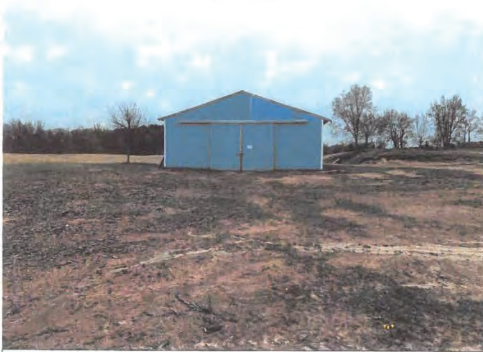
Picture 1 – Front of Larger Pole Barn Looking South.
