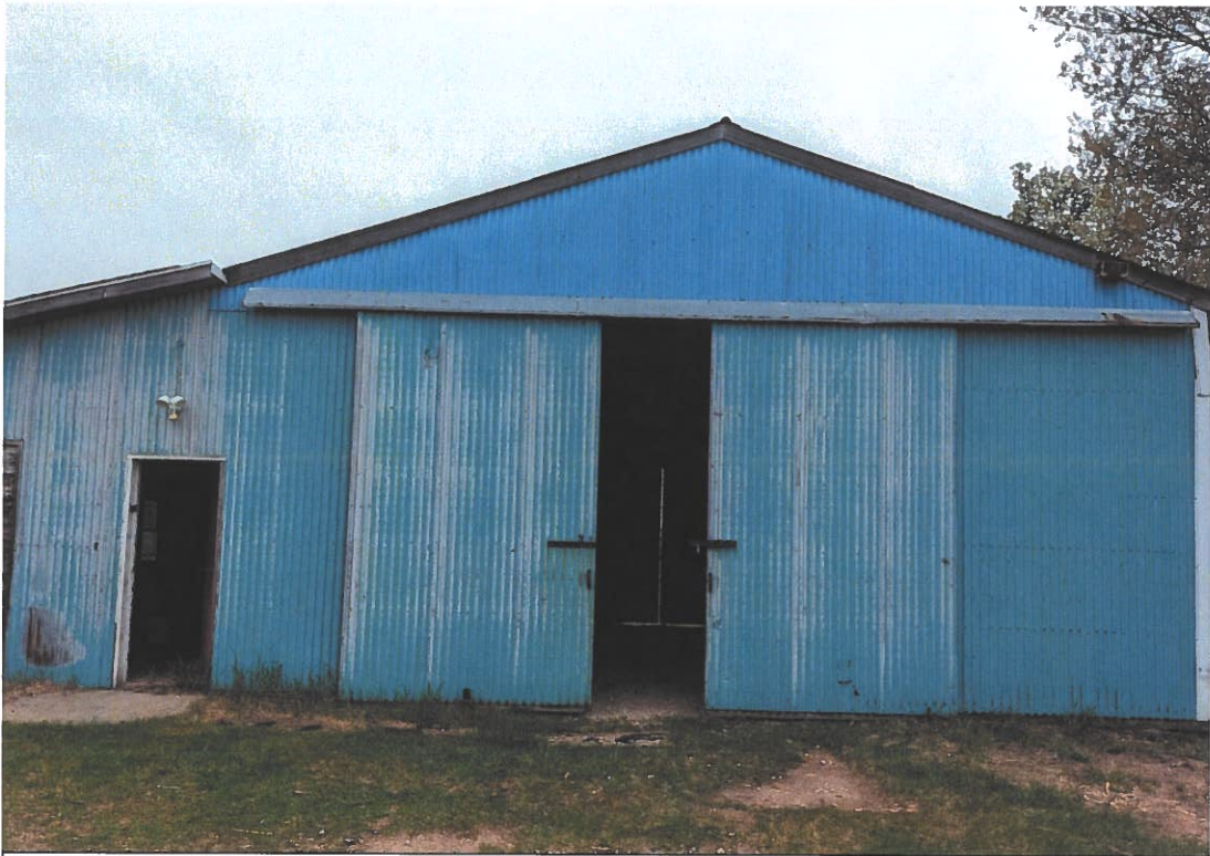
Picture 10 – Front of Smaller Pole Building Looking West
