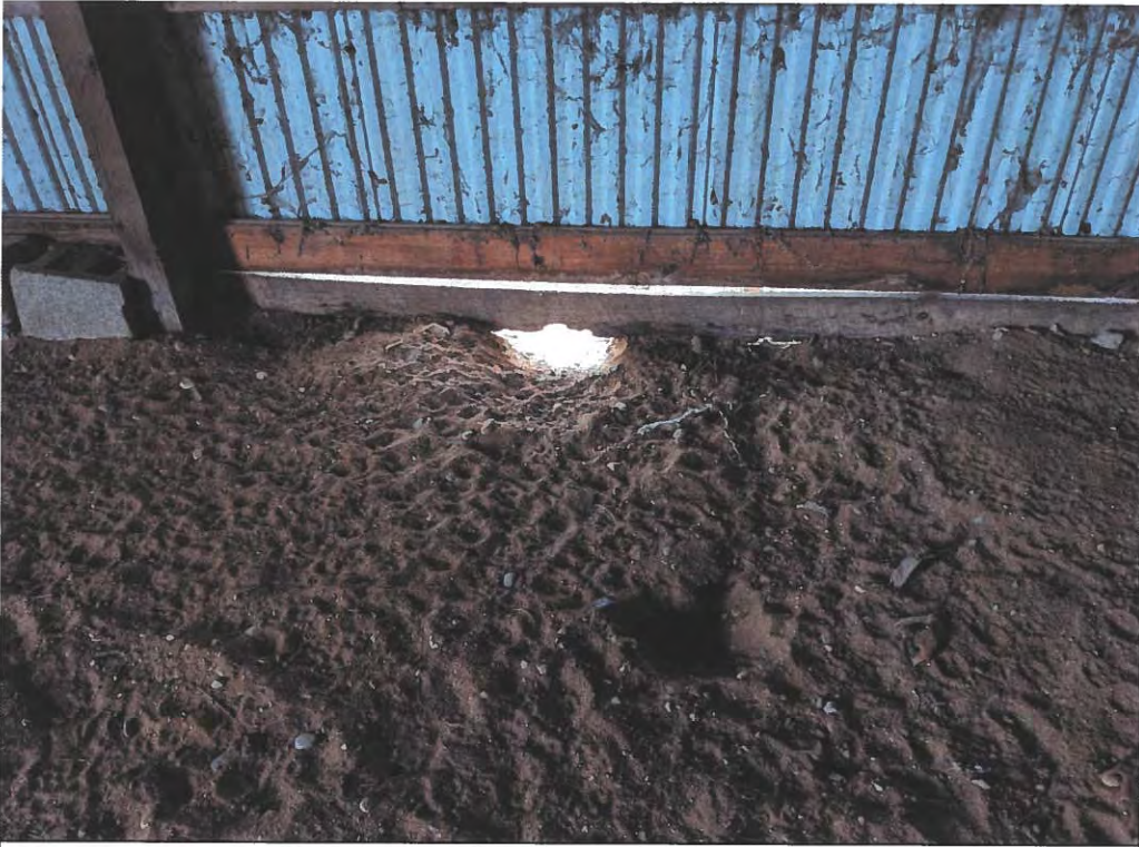
Picture 7 – Animal Entrance and Dens in Larger Pole Building
