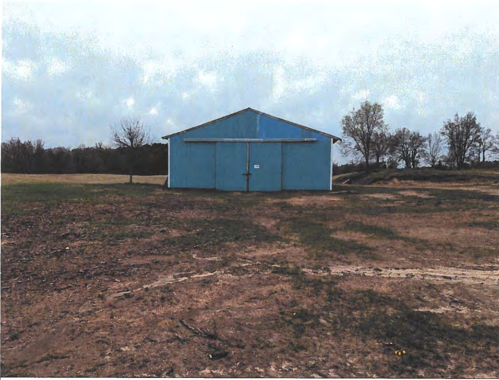
Picture 1 – Front of Larger Pole Barn Looking South.
