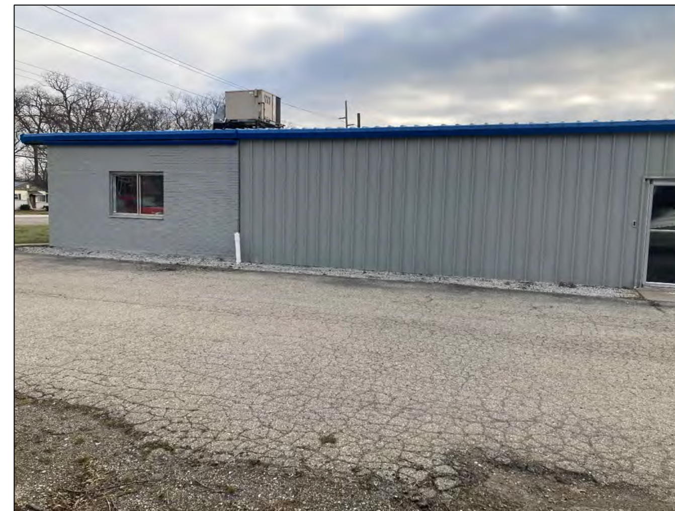
WEST BUILDING ELEVATION NORTH END
