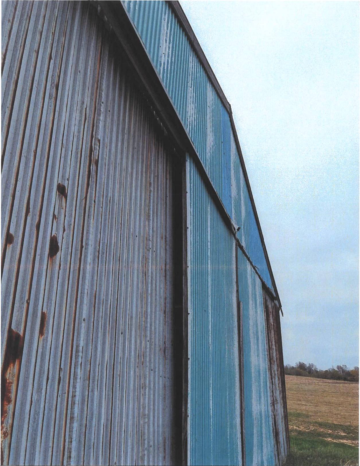
Picture 9 – Large Gaps Between Sliding Doors and Walls on Rear of Larger Pole Building
