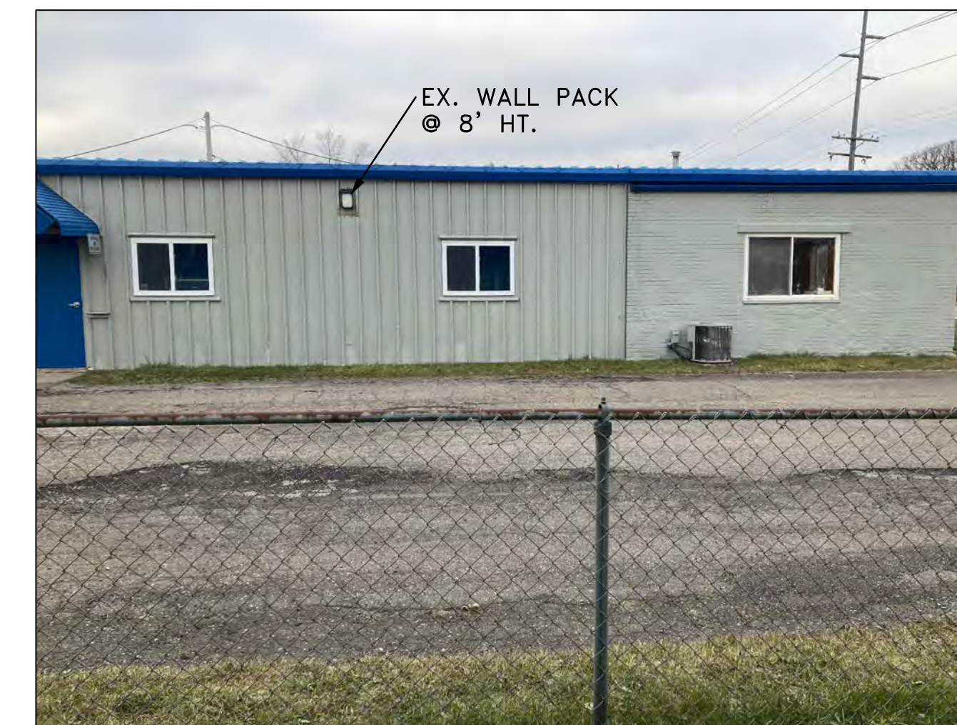
EAST BUILDING ELEVATION NORTH END
