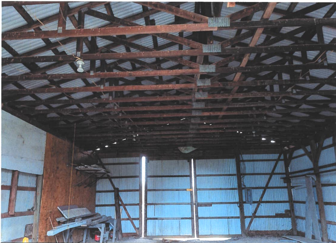
Picture 11 – Interior Smaller Pole Building Looking West
