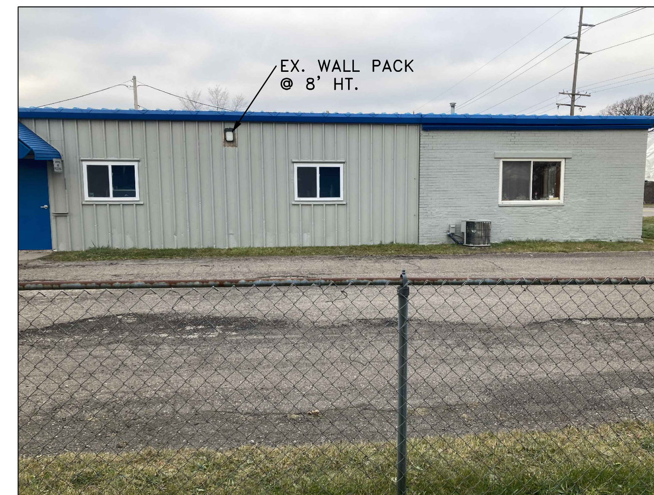
EAST BUILDING ELEVATION NORTH END
