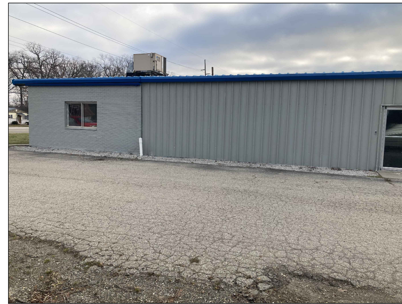
WEST BUILDING ELEVATION NORTH END
