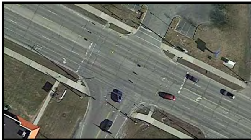
Figure 6: Grand River Avenue & Grand Oaks Drive Intersection
