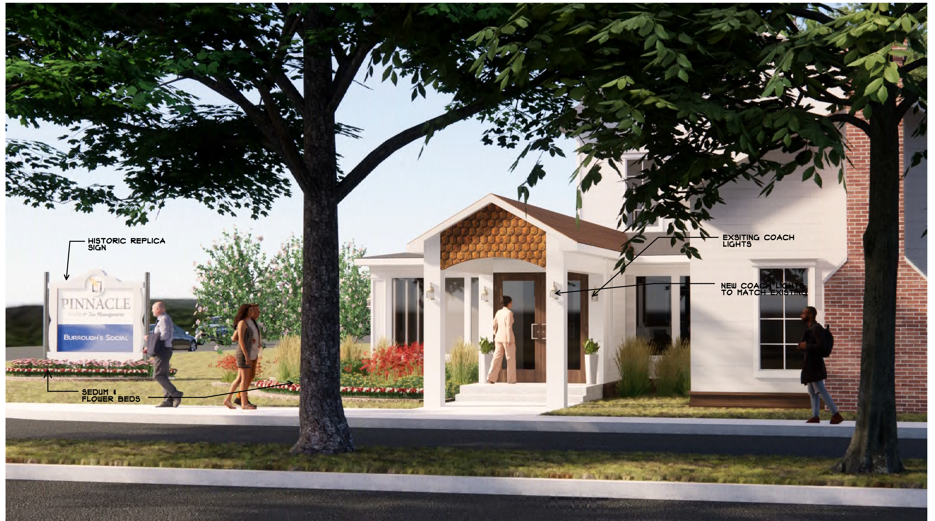
VIEW OF ENTRY FROM ENTRY DRIVE
