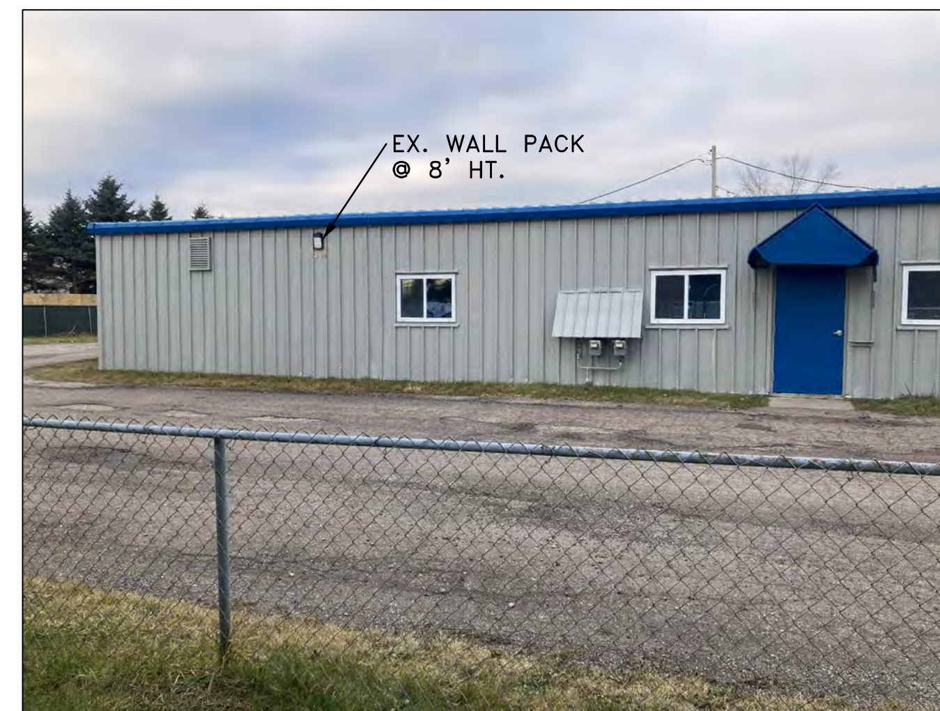
EAST BUILDING ELEVATION SOUTH END
