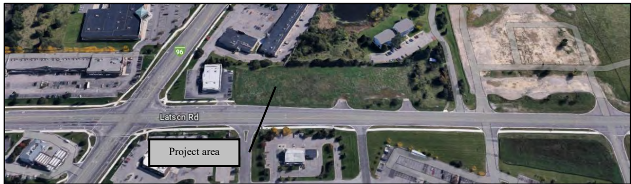
Aerial view of site and surroundings (looking east)
