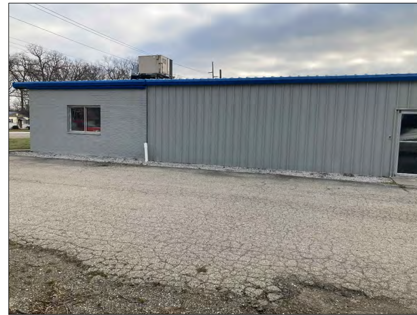
WEST BUILDING ELEVATION NORTH END
