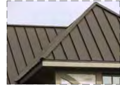
M-4: Standing Seam Metal Roof Manuf: Pac-Clad Color/Finish: Matte Black
