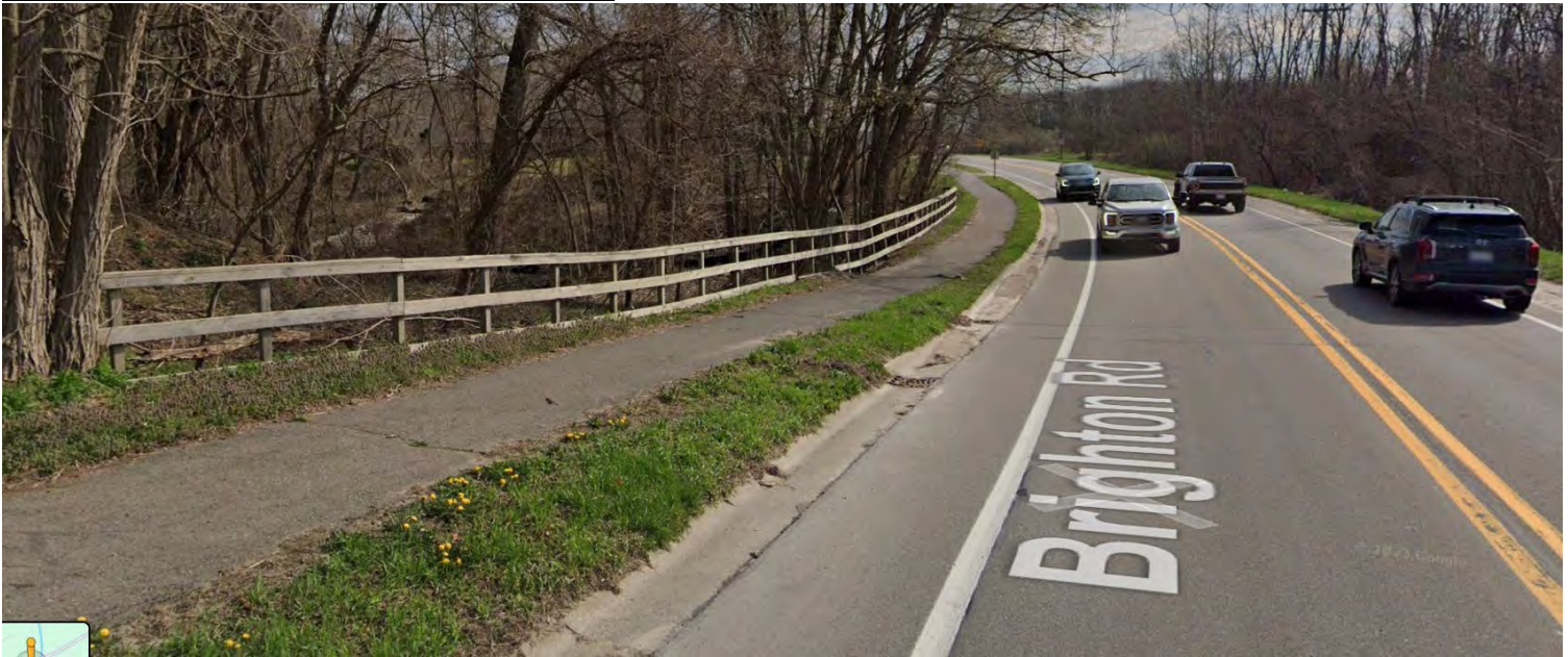
North side of Brighton Road – West of Bauer:
