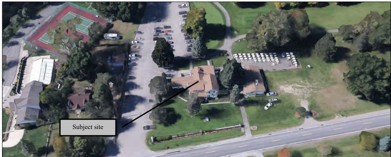
Aerial view of site and surroundings (looking north; prior to demolition)
