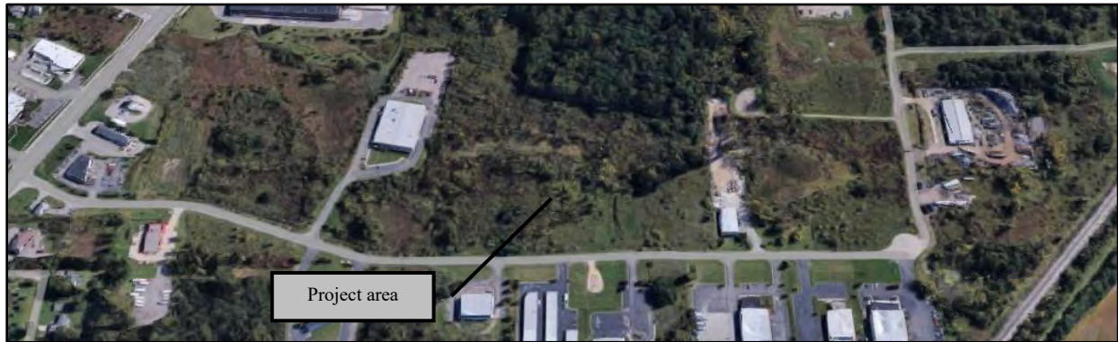
Aerial view of site and surroundings (looking east)
