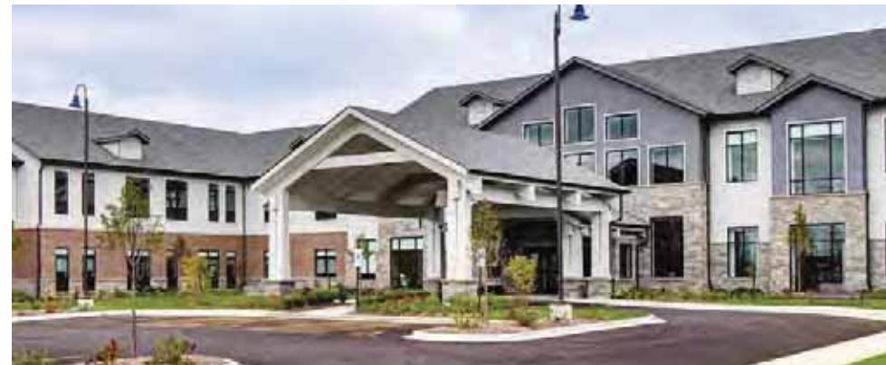
2.5-story attached special care facility
