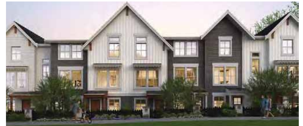
Stacked walk-up flats with rear-loaded parking
