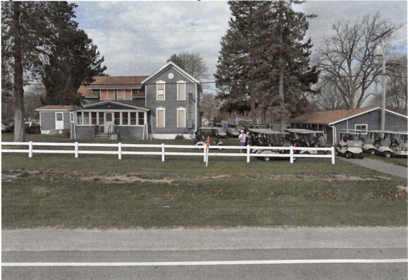
Figure 3 - Street View of Old Clubhouse and Storage/Maintenance Building, April 2023
