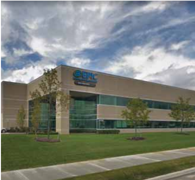
EPIC Equipment and Engineering, Shelby Parkway Corporate Park
