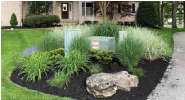
Utilities screened by shrub plantings
