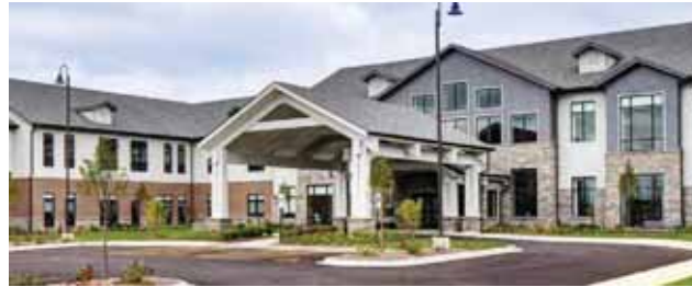
2.5-story attached special care facility
