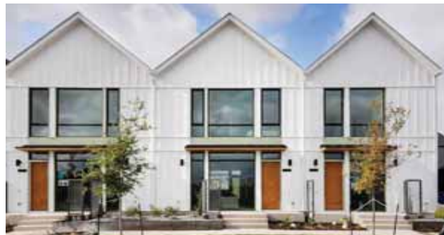
2-story walkup townhomes
