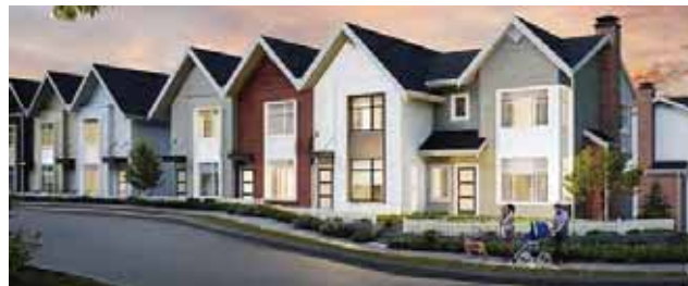
2-story walkup townhomes
