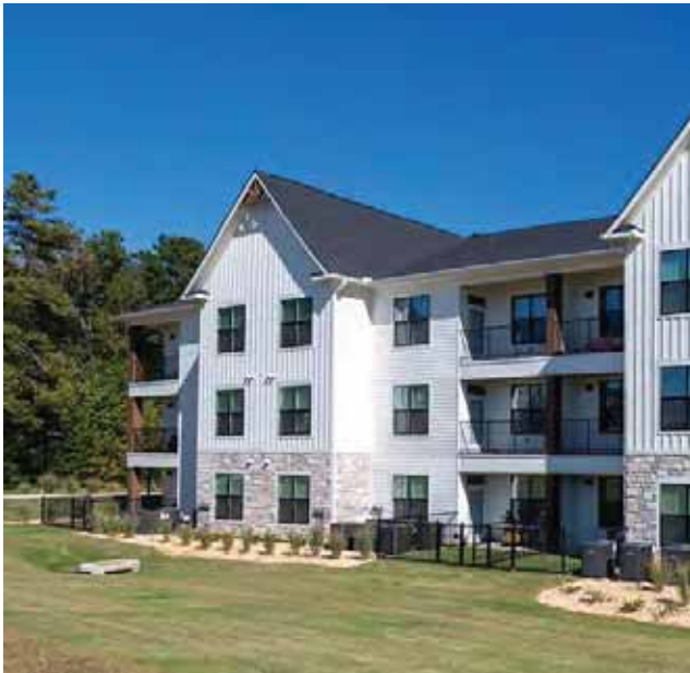
Stacked flats with rear open space
