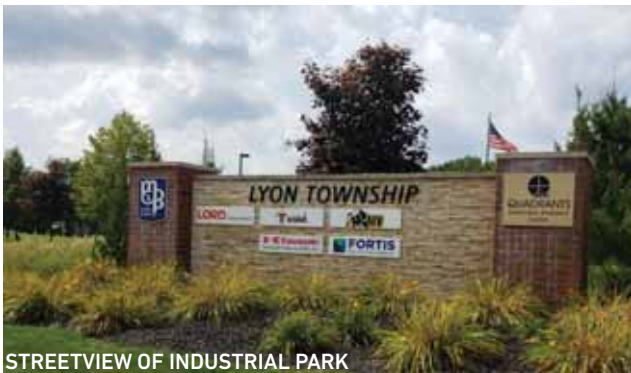
STREETVIEW OF INDUSTRIAL PARK
