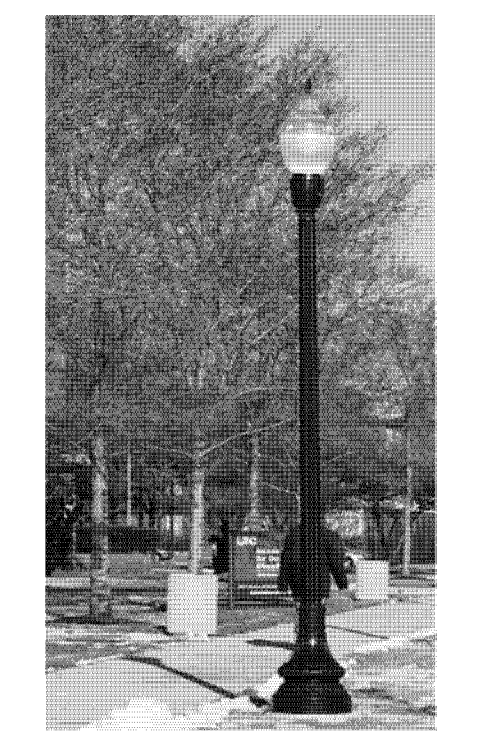
A decorative pole and light (5-CONDITION) DECORATIVE BLVD. ISLAND SITE FIXTURE LIGHTS AND ALUMINUM POLE.
