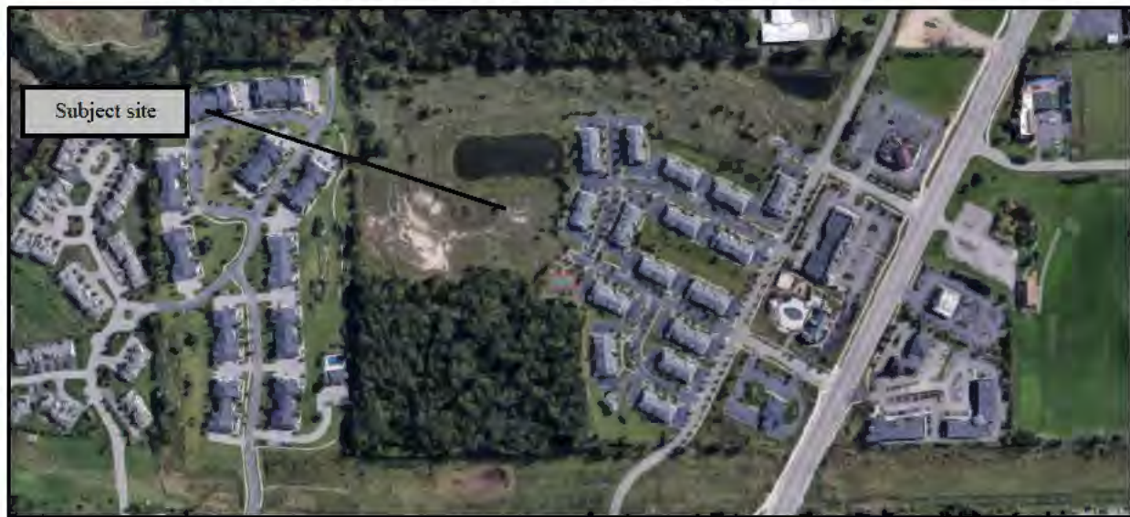
Aerial view of site and surroundings (looking east)
