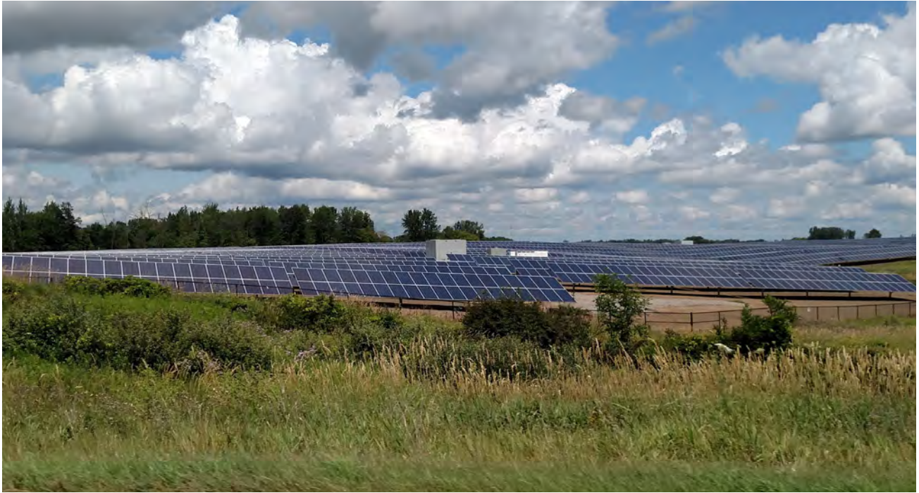
Lapeer Solar Park. Photo by Bradley Neumann.
