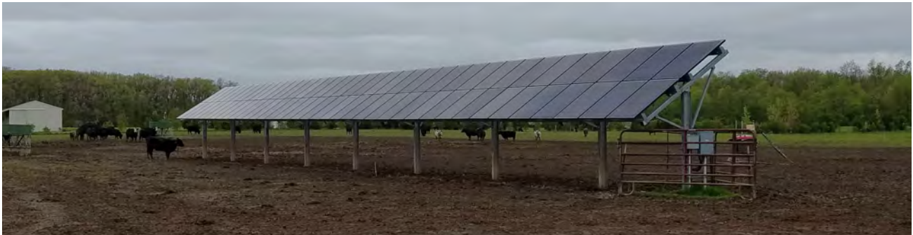
Ground-mounted SES feedlot. Photo by M.Charles Gould.
