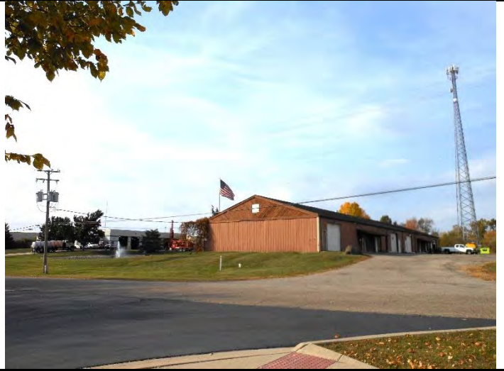
West – Industries on Sterling Drive
