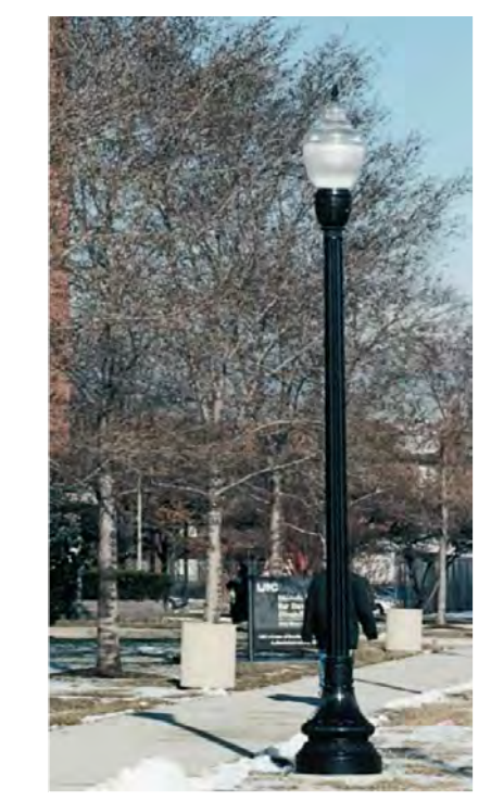
A decorative pole and light (5-CONDITION) DECORATIVE BLVD. ISLAND SITE FIXTURE LIGHTS AND ALUMINUM POLE.
