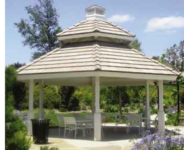
F gazebo feature (1-CONDITIONS) STICK BUILT OR KIT FORM. TO BE BUILT BY MANUFACTURER STANDARDS
