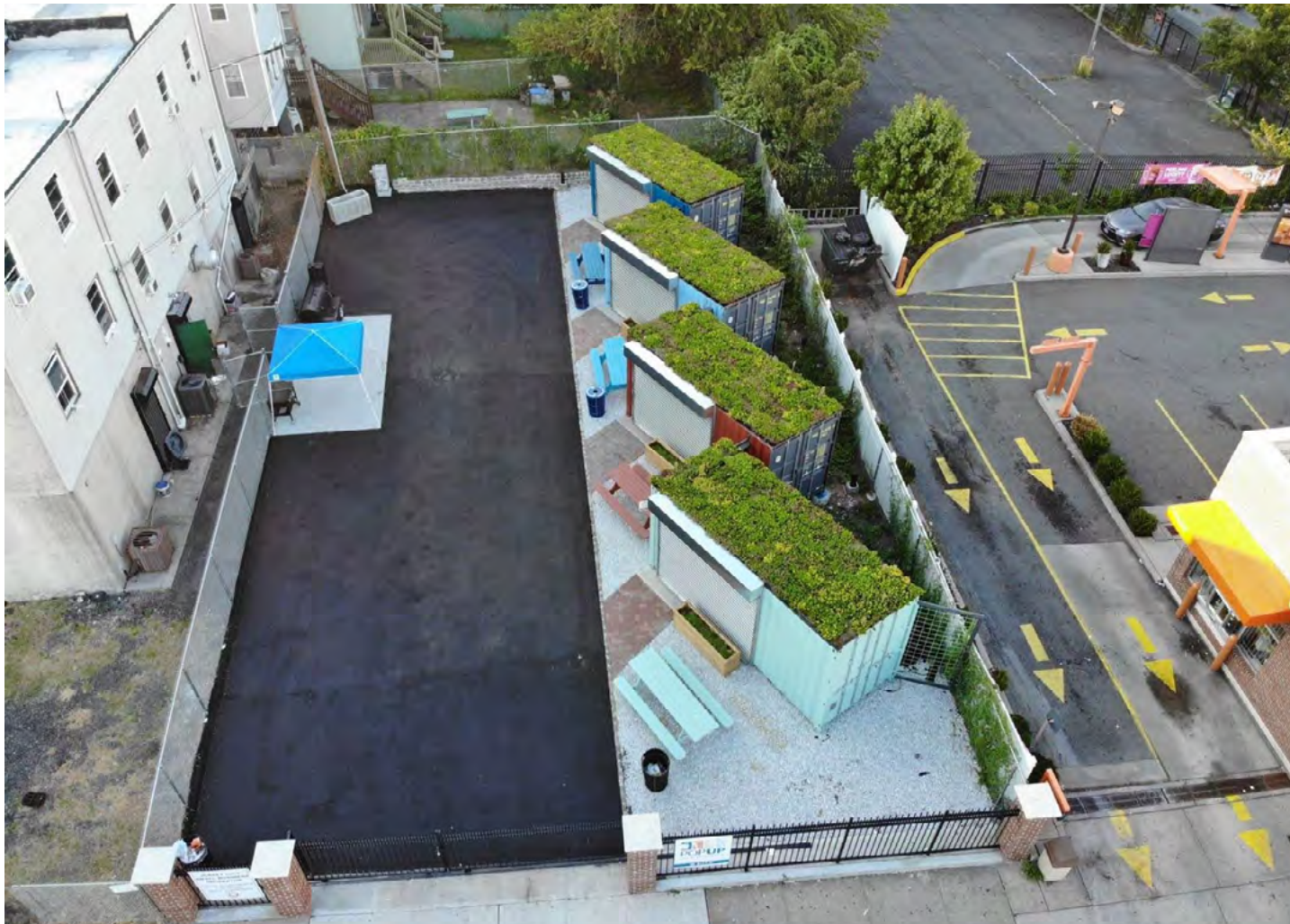
Container Village 342 MLK Drive Bergen Lafayette Jersey City NJ. Source: Jersey City
