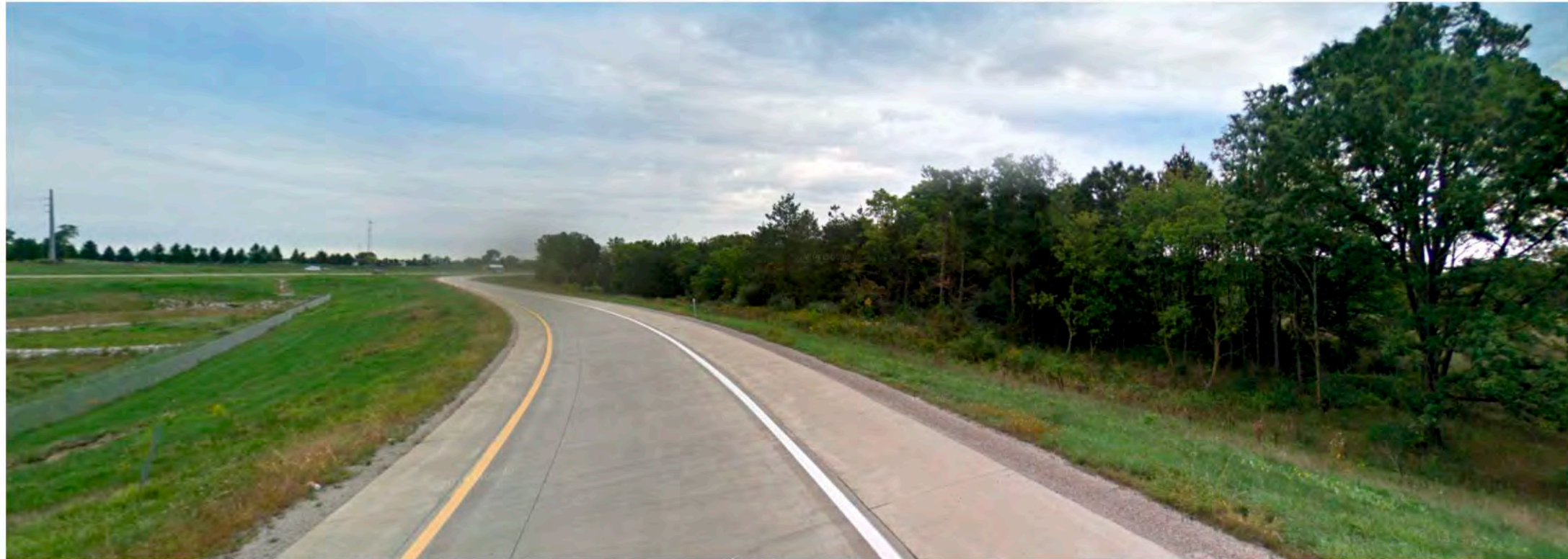
SUMMER VIEW - CURRENT CONDITION
