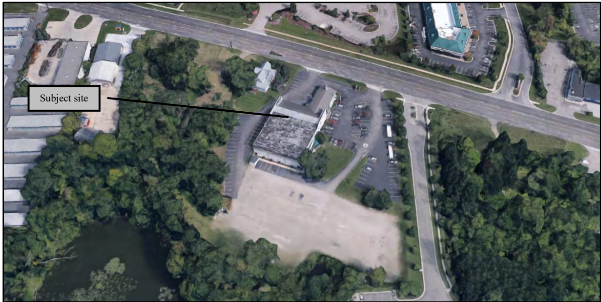
Aerial view of site and surroundings (looking north; prior to recent remodel/expansion)
