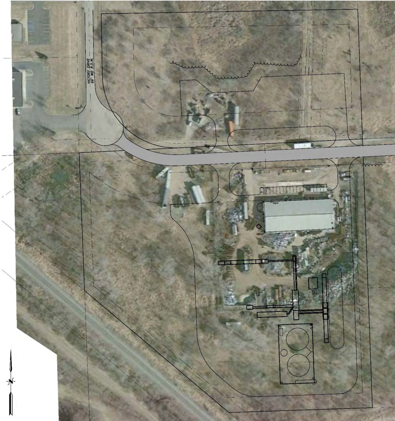
FIGURE 2 PHOTO DEPICTING SITE IMPROVEMENTS NOT TO SCALE
