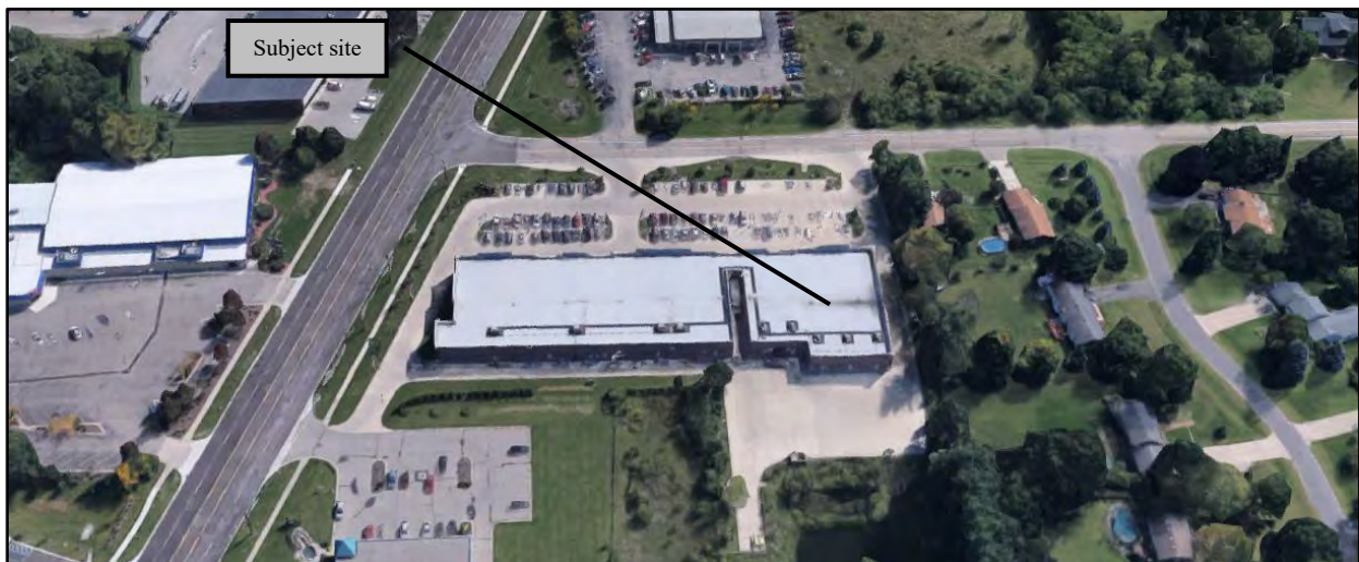
Aerial view of site and surroundings (looking east)
