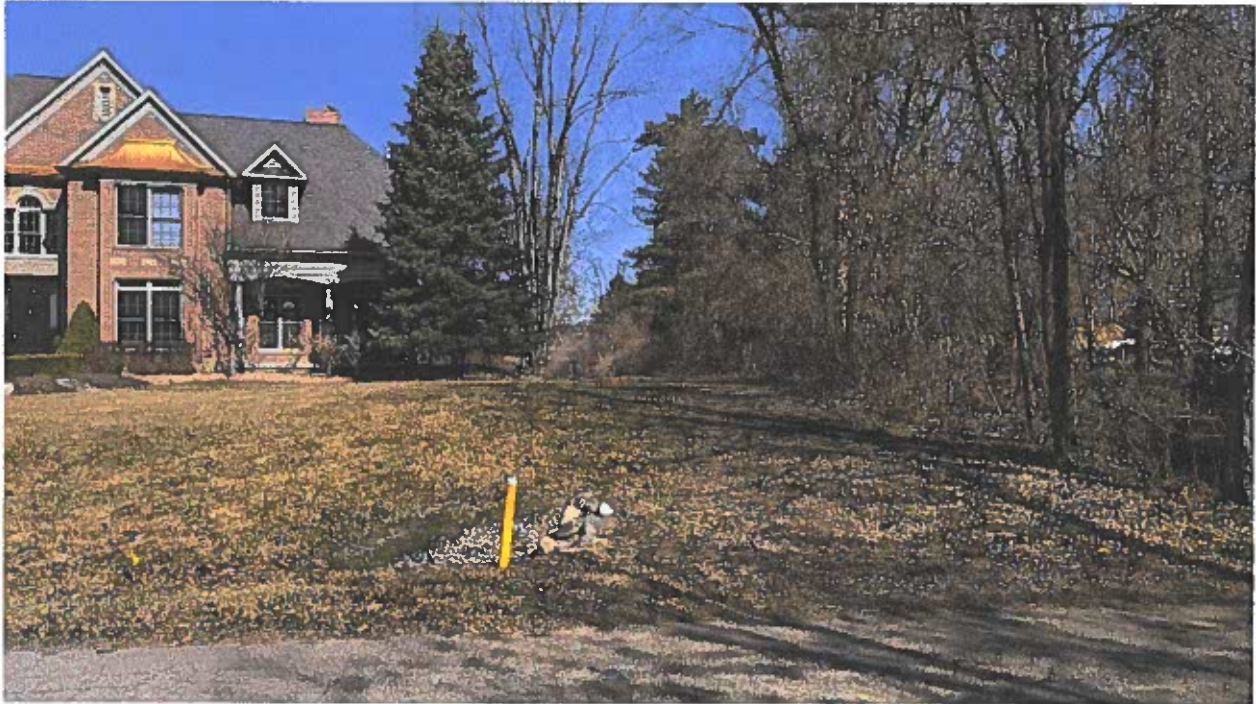
The image above is seen as standing in front of the residence at 7873 Shores Pointe Drive, looking North towards the property showing that the retaining wall will not be visible given the difference in elevation from the street to the property.
