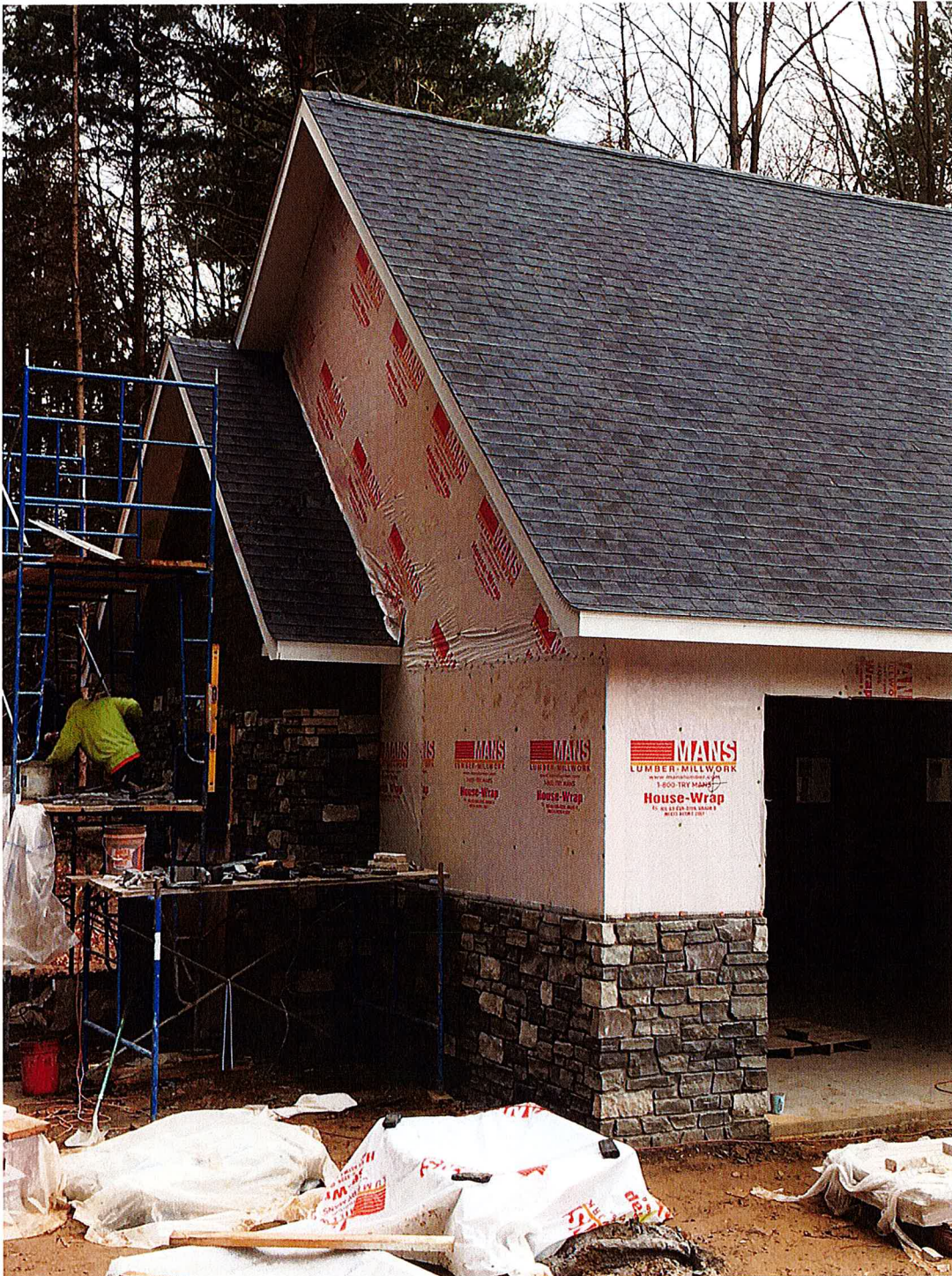
Detached out building located at 4320 Ridge Lake Court.
