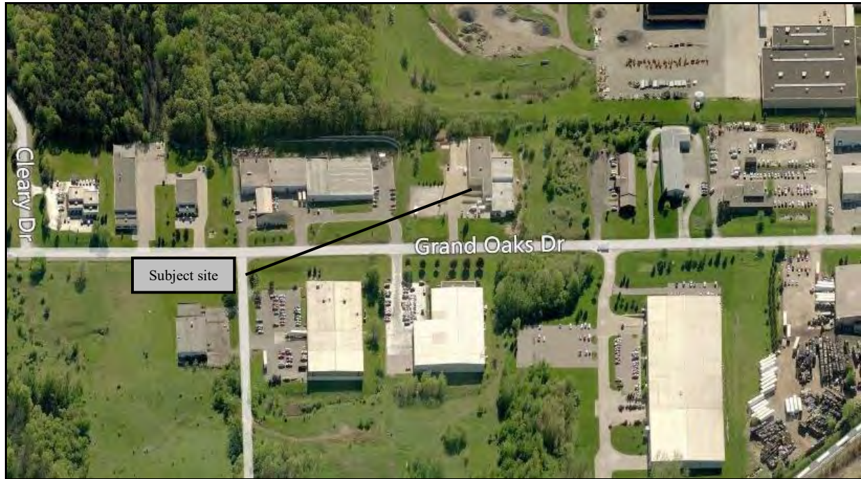
Aerial view of site and surroundings (looking east)
