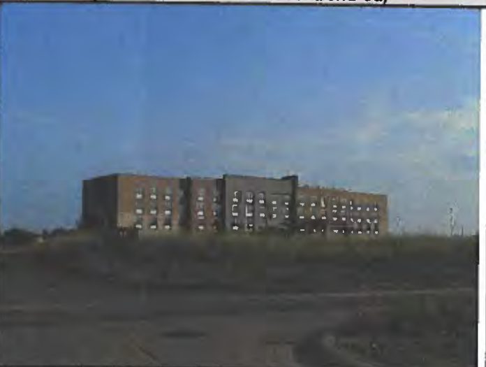
North of I-96 interchange on west side of Latson
