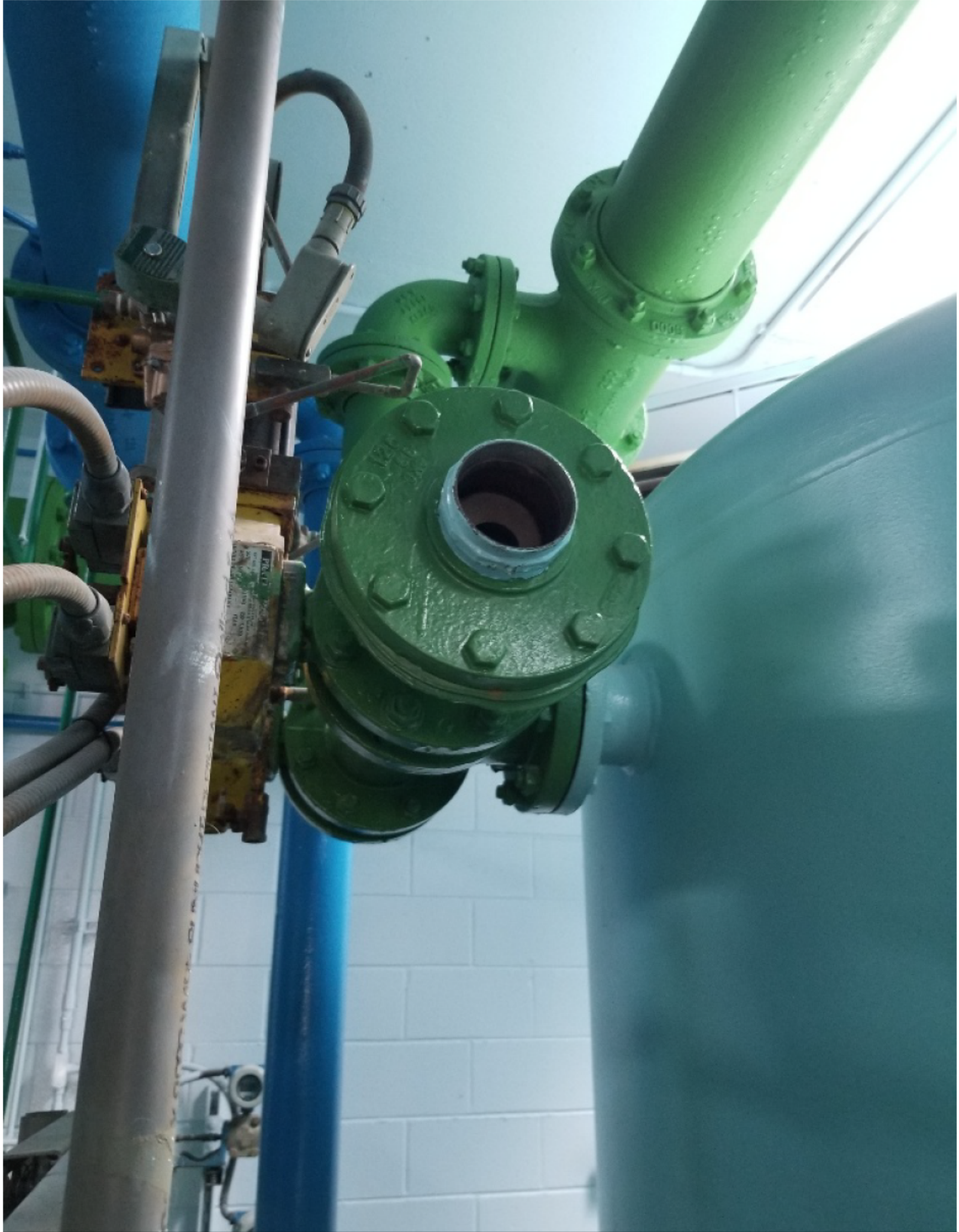
Backwash Outlet with Piping Removed
