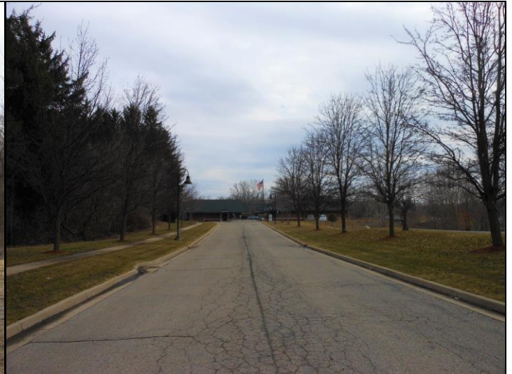
SITE – Northern Developed Portion
