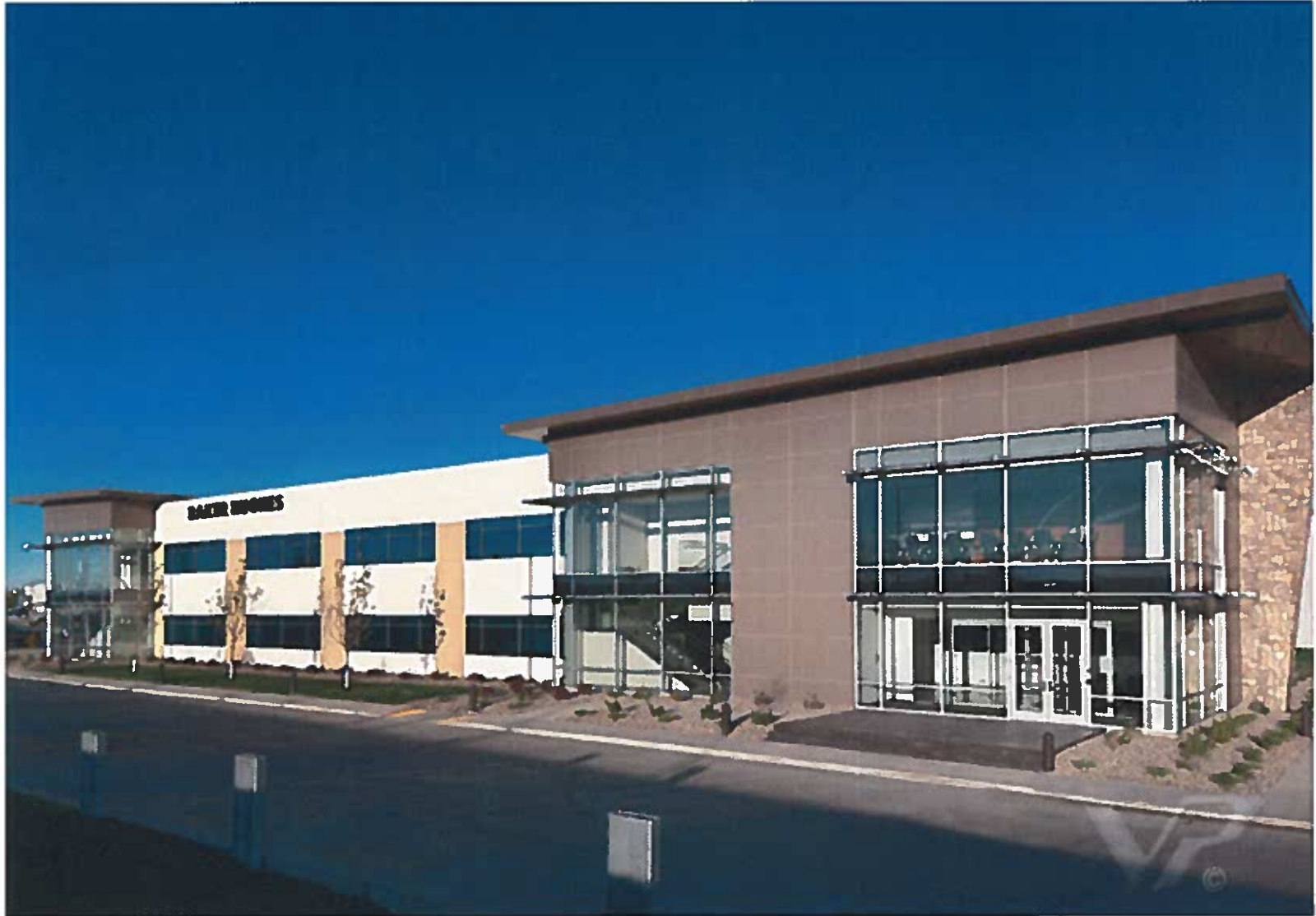
Baker Hughes Joint Facility Administration Building Williston, ND - Crossland Construction Company
