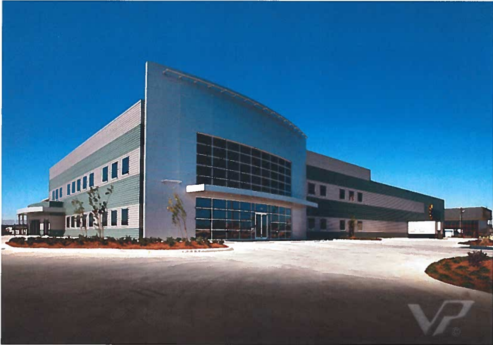
Kossen Equipment - Richland, MS - Peoples Construction Corp.
