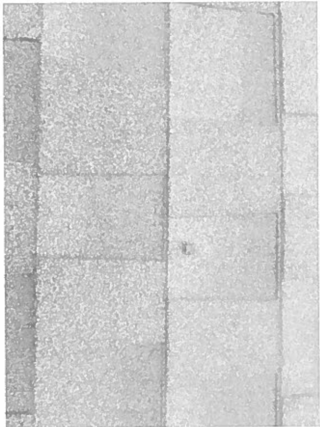
Additional backed-out nail example.
