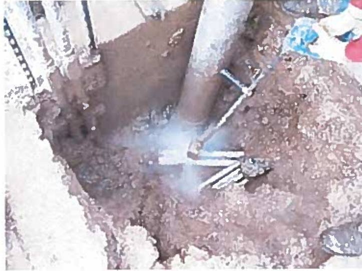
Example of Safe and Effective Hydroexcavation to Expose Utilities
