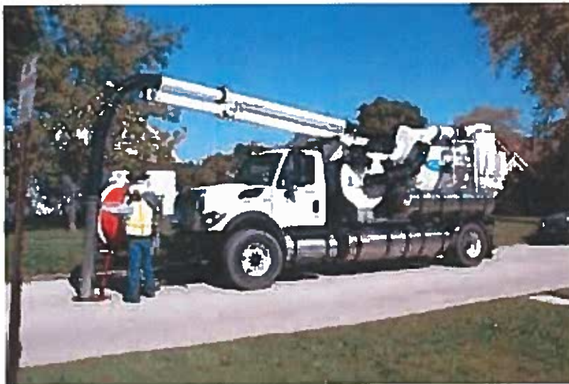
Sanitary Sewer Cleaning
