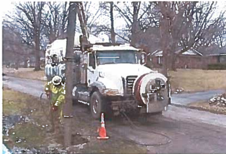
Hydroexcavation Utilizing Vector Truck
