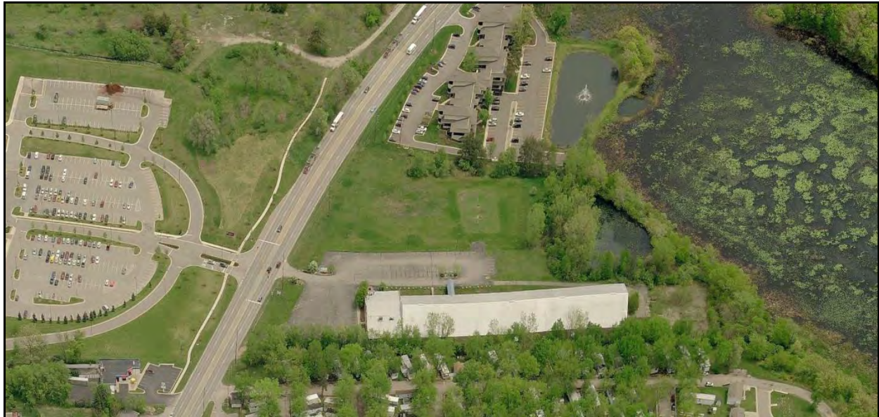
Aerial view of site and surroundings (looking east)
