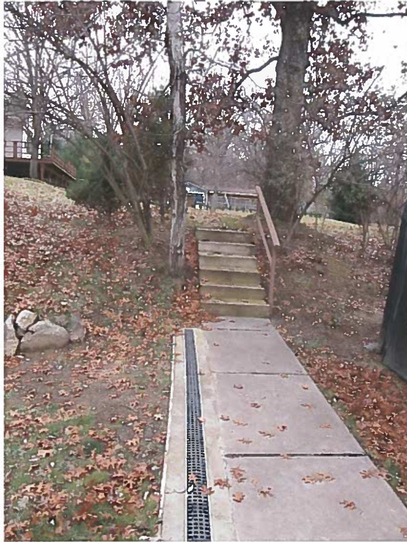
South front view from existing Structure
