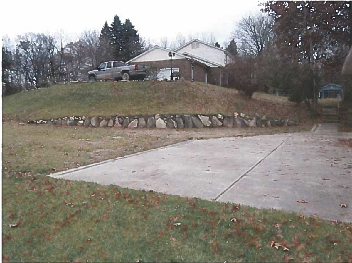
South front view of existing Structure
