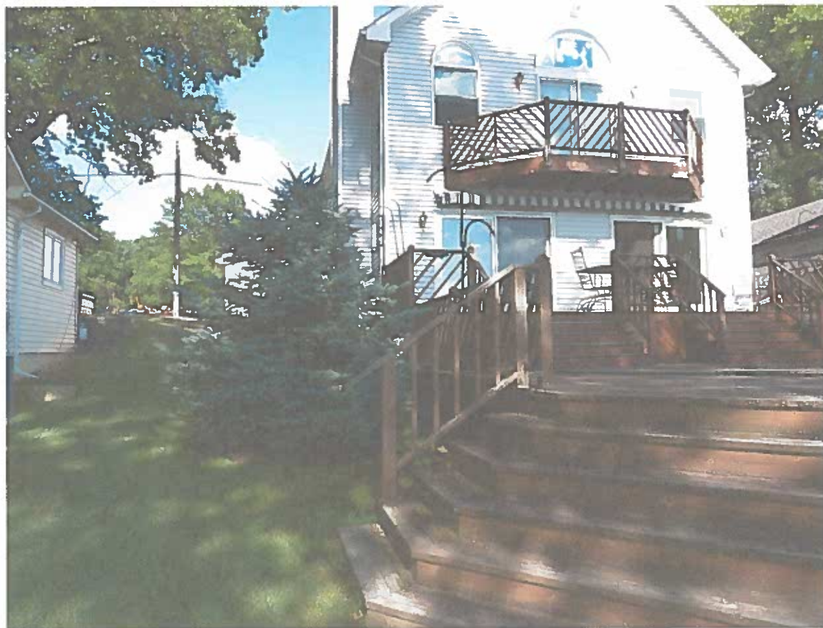
Alignment of current deck footprint with sides of house, showing existing tree on north side.
