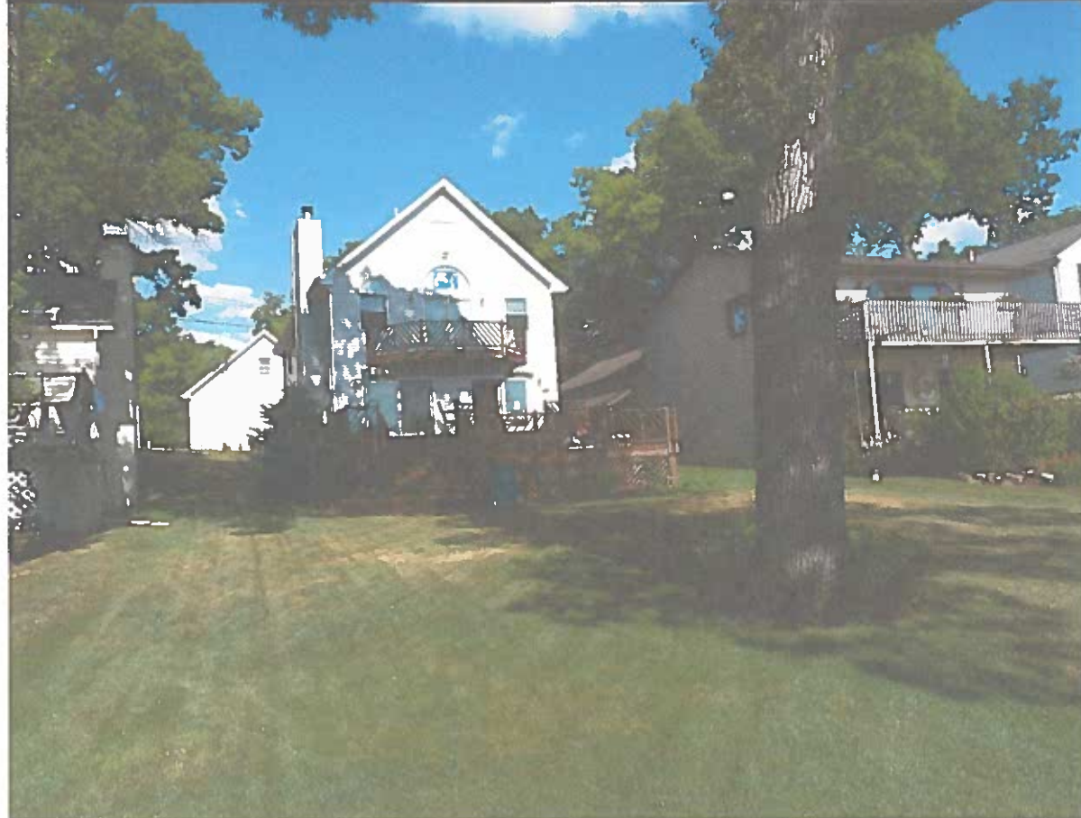
Top: double door wall in relation to 2 levels of lower deck. Existing deck measures 27 ft out from house (not including steps to lawn which measure additional 6 ft), deck sides match up with house sides at 26 ft 3 in, with 2 ft to south lot line. Bottom: from seawall, shows setback from lake, which is 60 ft from seawall to deck (not including steps to ground), or 87 ft to house.
