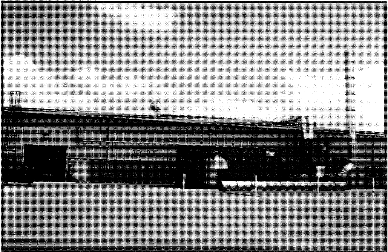
View of Drum Yard inside
