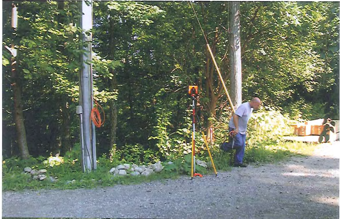
Survey work done after fence posts remove from 6483 Forest Beach
