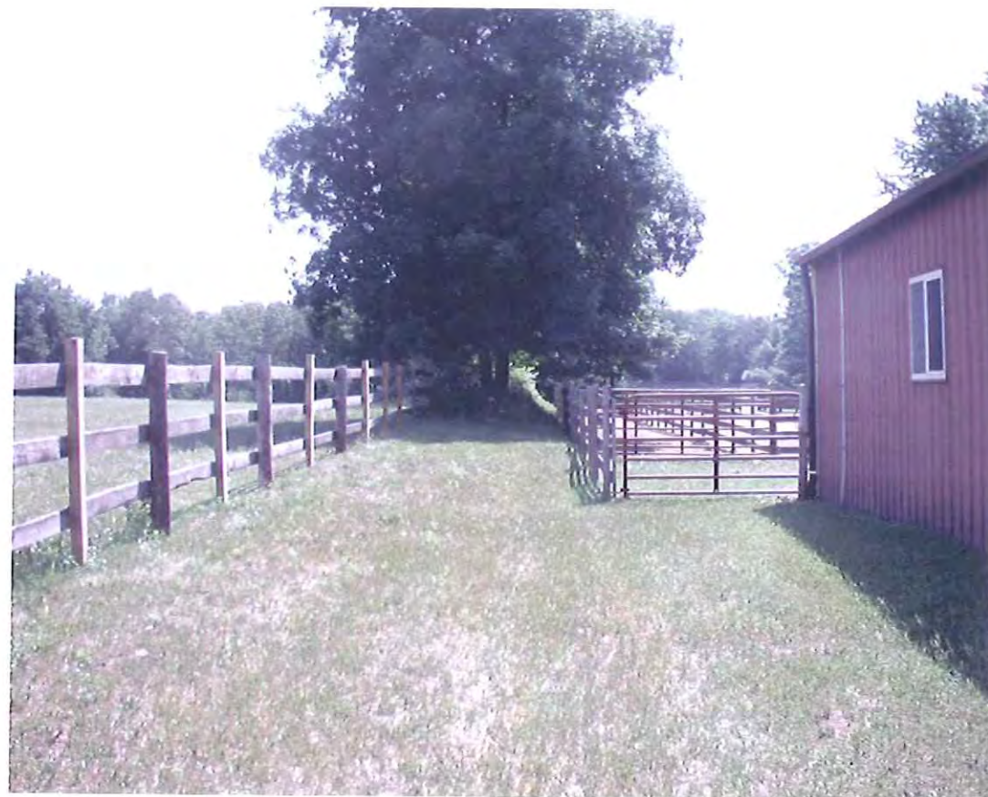
NORTHEAST CORNER OF EXISTING BARN
