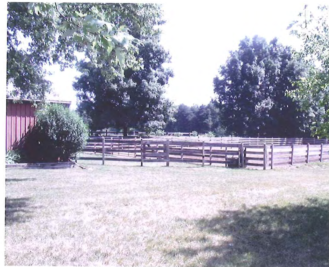
SOUTHEAST CORNER OF EXISTING BARN
