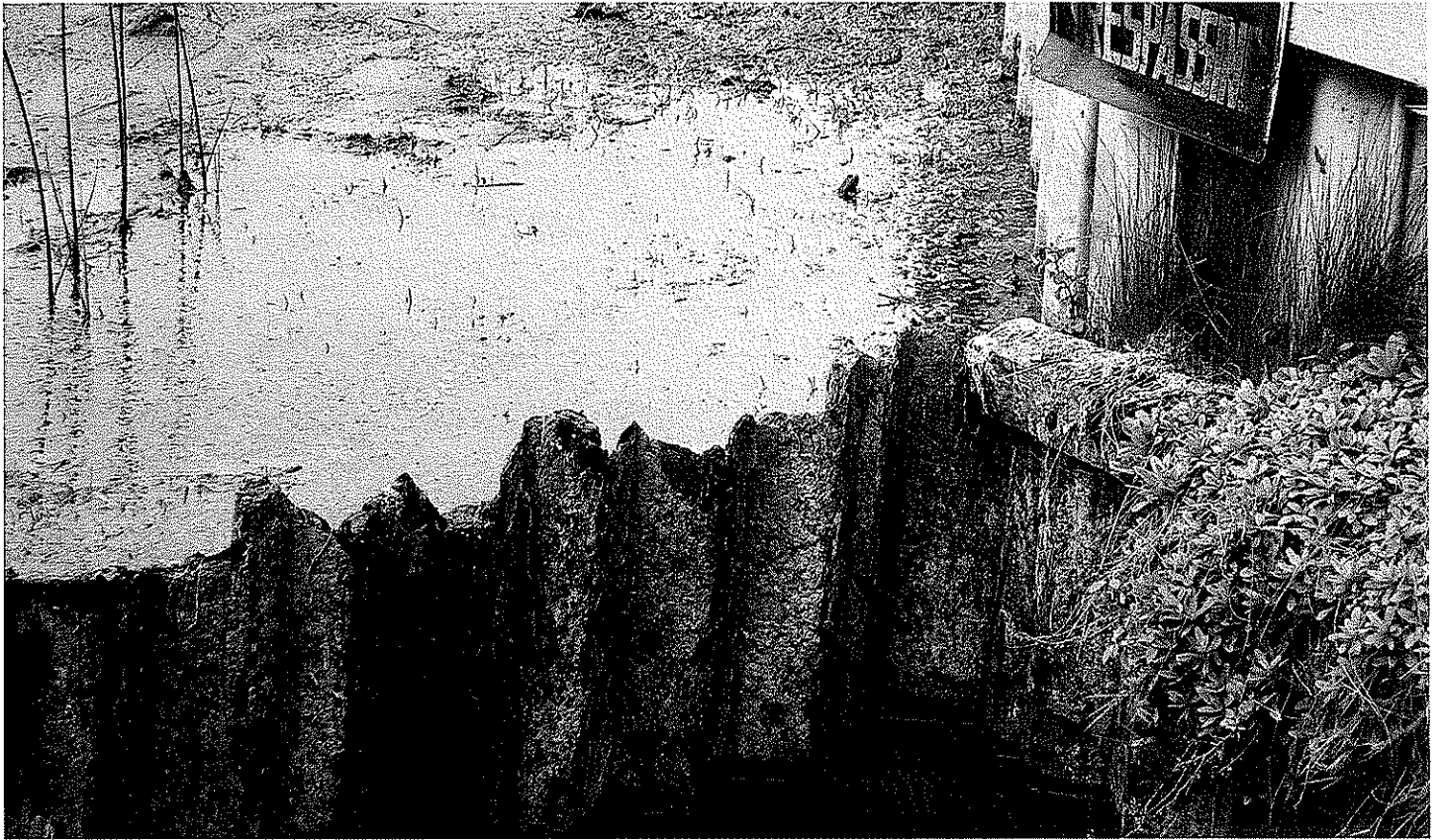
Lake Chemung Dam weir deterioration.
