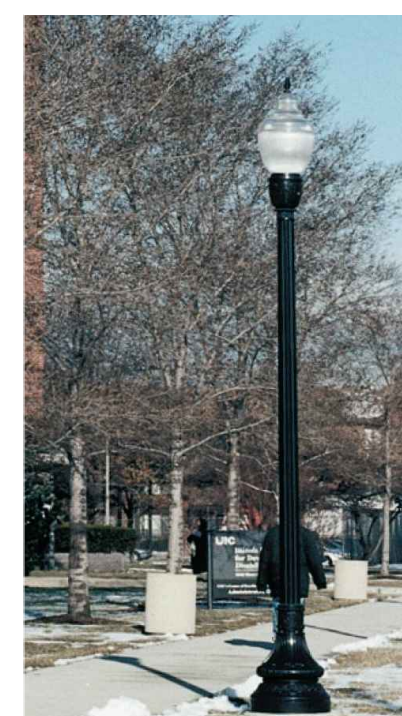
A decorative pole and light (5-CONDITIONS) DECORATIVE BLVD. ISLAND SITE FIXTURE LIGHTS AND ALUMINUM POLE.
